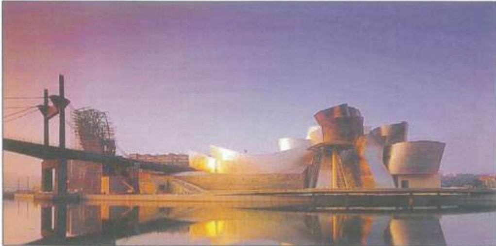
Plate 3: Frank Gehry, b. 1929, Canadian, Guggenheim Art Museum , on the banks of the Nervion River, Bilbao, Spain, 1997, steel frame, titanium sheathing, 50 m. height.
